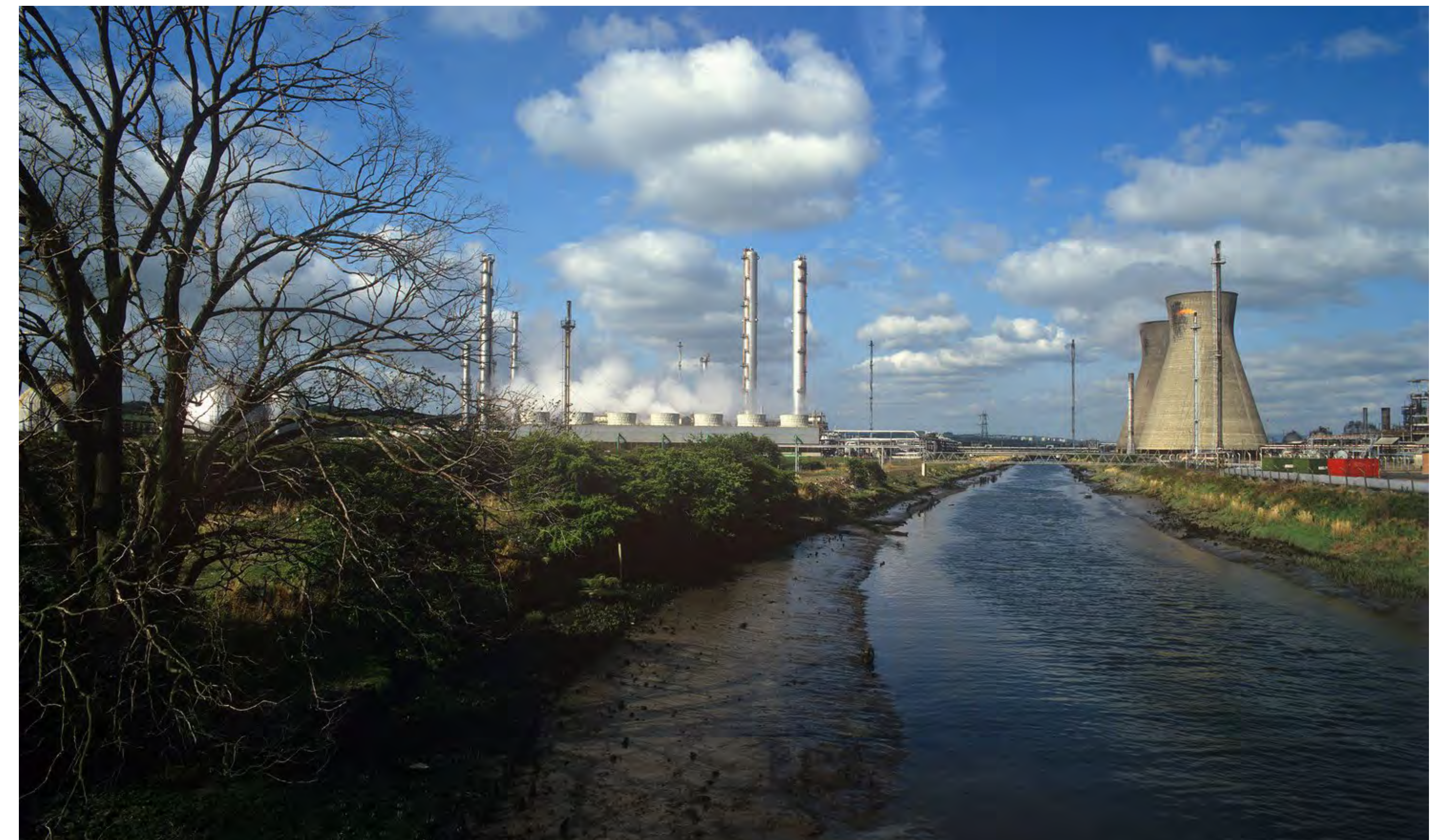
Photo looking west from the Grangemouth Road bridge crossing the River Avon - the site is on the left hand side.
